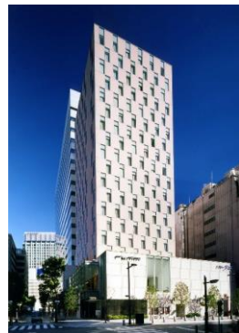
Toho Theatre Creation Bldg. (Tokyo) Property use: Theater, Hotel
